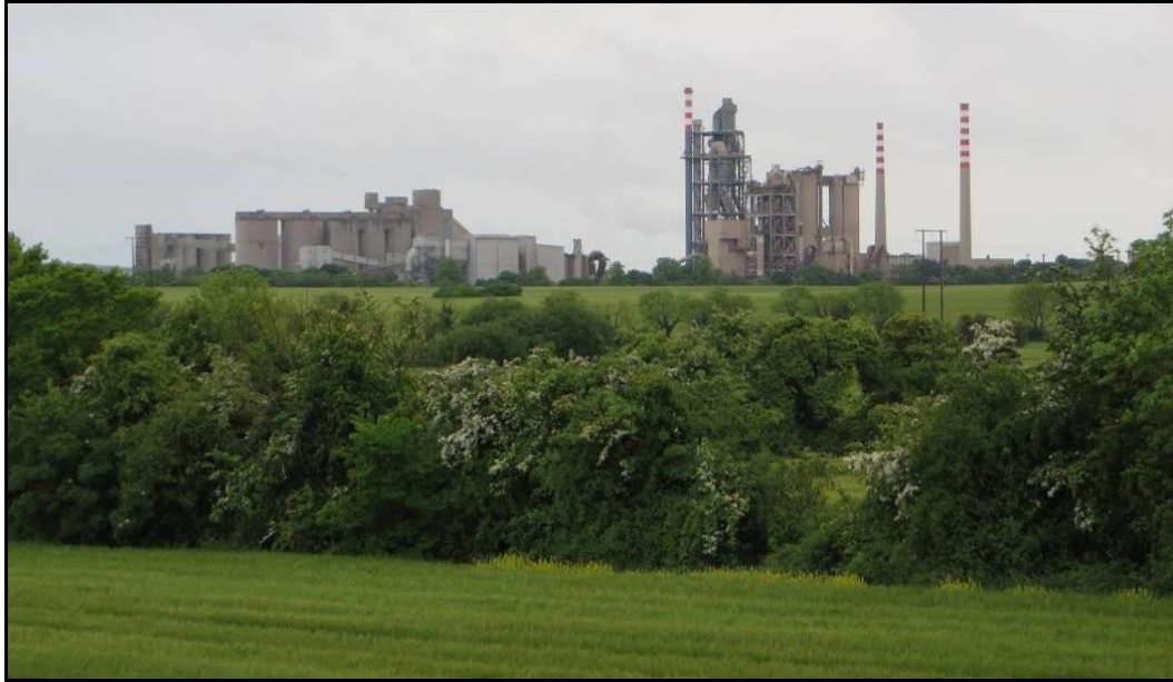
Plate 7 Irish Cement plant at Platin, Duleek, Co. Meath.
